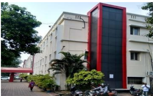
Figure 2 Secha Sadan building
